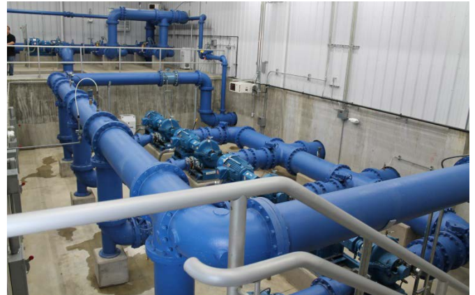
Bartlett Pumping Station
